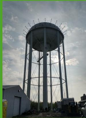
Notice a difference in the skyline in your neighborhood? Our Bethel St. water tower is getting a makeover! The brackets as shown are tarp containment brackets. When it's time, a tarp will be placed over the water tower to mitigate debris from sandblasting and paint overspray on neighboring properties and these brackets will help hold the tarp in place. Follow our Facebook page for more updates on the progress of the water tower makeover and to see the final product!
